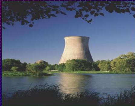
Nuclear Power Plant
